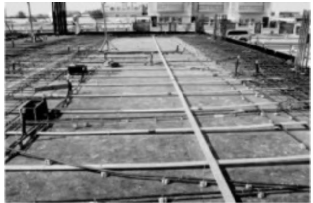
Figure 1: Typical Layout of Bonded System
