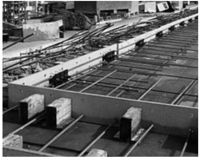
Pulling anchors for post-tension cables
