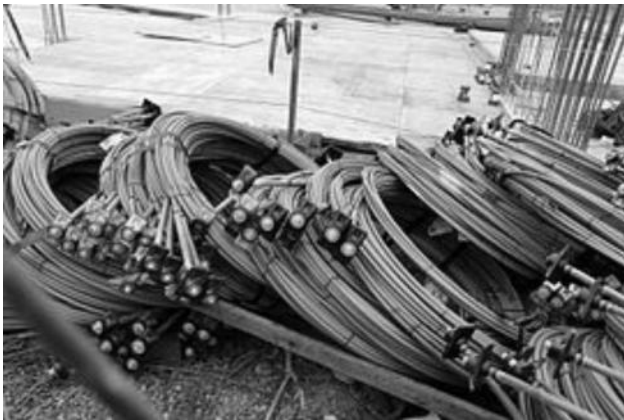
Rolls of post-tension cables
