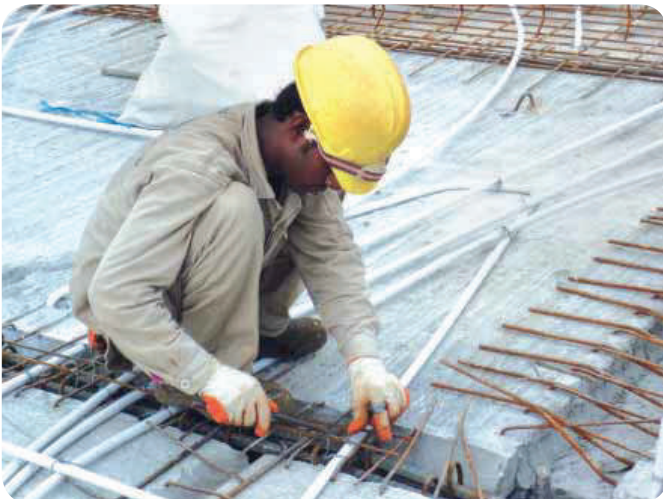
Securing of conduits to re-bars
