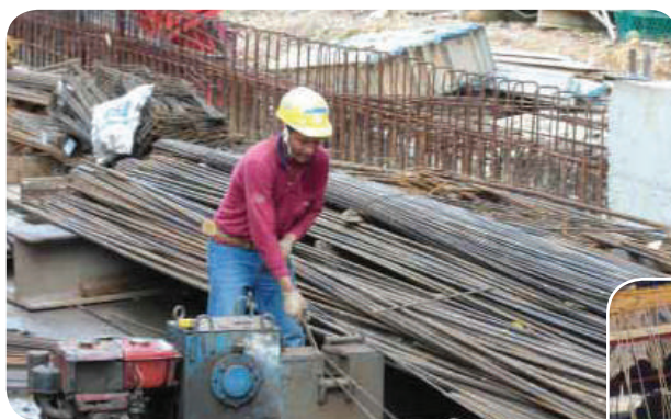
..... Cutting of re-bars ..... to required length
