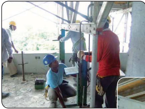
Lowering down the table formwork
