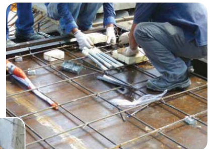
Securing of conduits junction box
