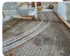
Fixing of top reinforcements and securing of conduits to ensure they are firmly in position before concreting
