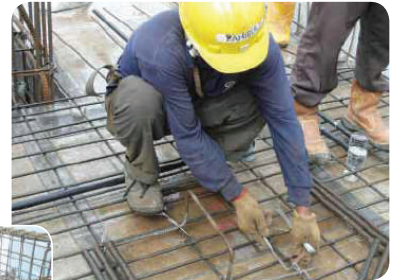
Fixing of re-bars using hand tool
