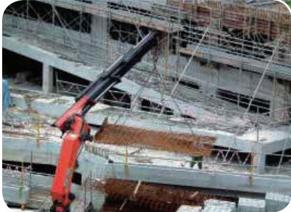
Transporting of prefabricated mesh to working area
