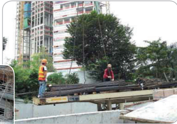
Transporting of re-bars to working area
