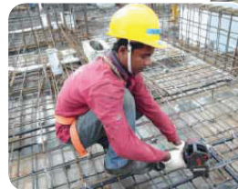
Fixing of re-bars using mechanical means
