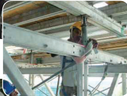
Securing lifting cable to formwork
