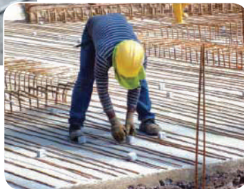
Placing of concrete spacer
