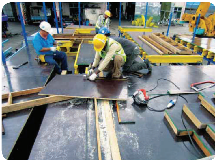
⋮ Placing of infill panel
