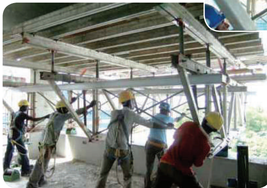
Shifting of table formwork out of building
