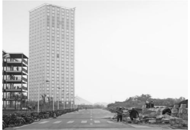
30-Story Steel Building
