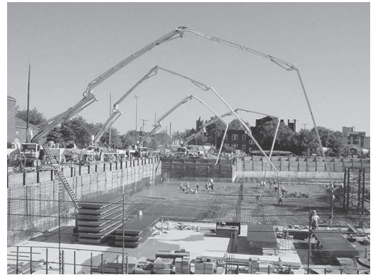
Fig.5.13 Boom placer in operation
