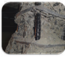
The Bond between Epoxy Coated Rebar and Concrete
