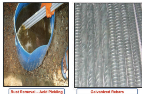
Rust Removal – Acid Pickling
