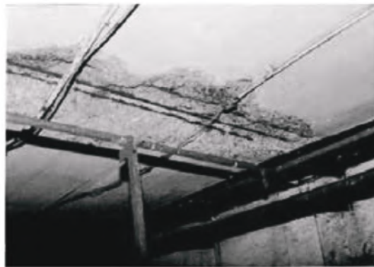
Fig. 7 Corrosion due to stray currents
