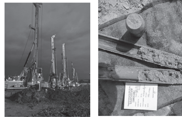
BORED PILES – Hydraulic Rotary Rig Piles
