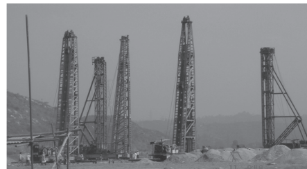
DRIVEN PILE RIGS
