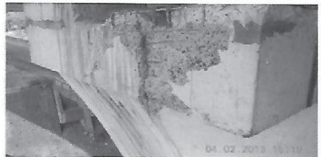
Fig. 8 : Cracks in the pier cap
