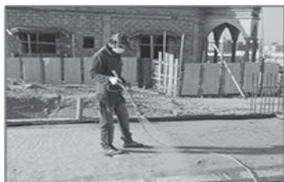
Anti-Termite treatment in foundation
