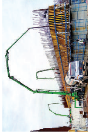
Concrete Boom Pump, S36 working at a bridge construction site
